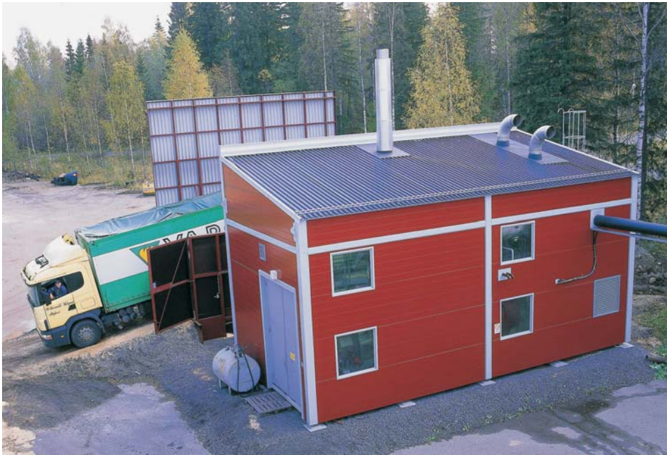
Figure 11. Ekotuli heating plant at Tikkakoski (Courtesy of Vapo Oy).
